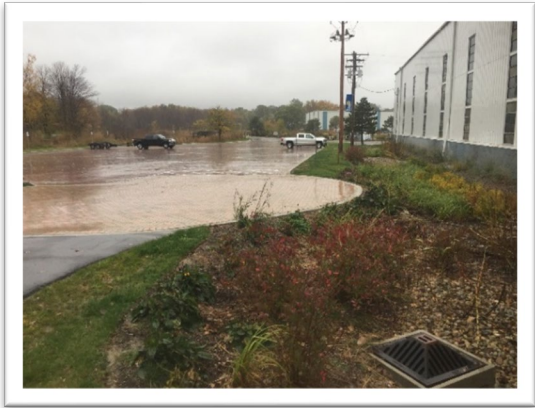
Permeable pavement with bioretention
