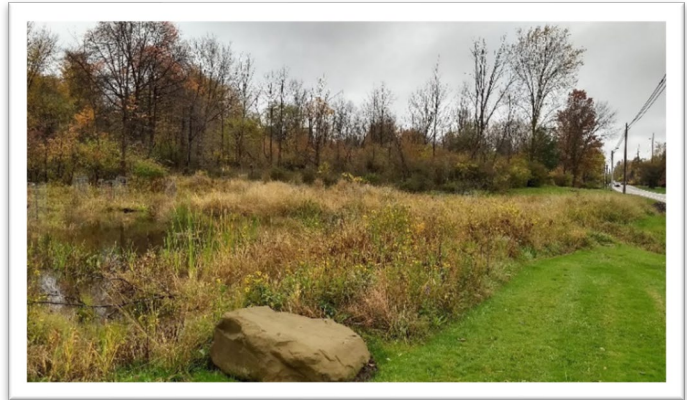
Wetland created to address excess stormwater
